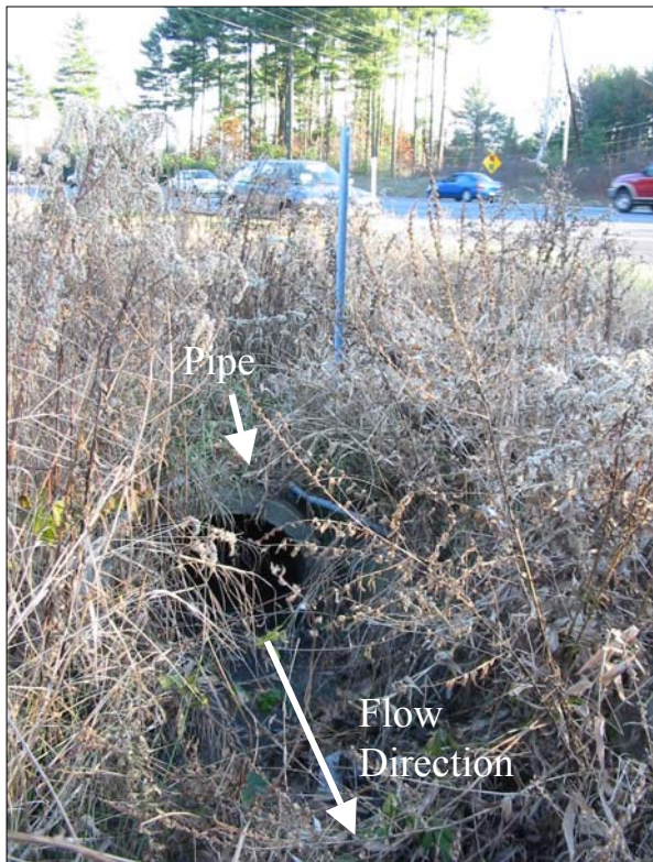
Figure 3-2. Route 101A 24” Discharge Looking Southeast Facing Road
