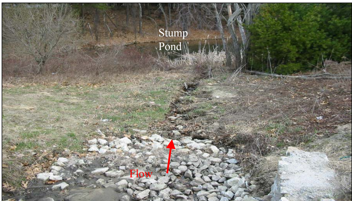
Figure 3-9. Route 101A Discharge to Stump Pond Facing Pond
