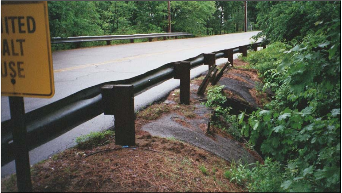
Figure 3-6. Asphalted bank Around Culvert of Craftsman Lane Bridge
