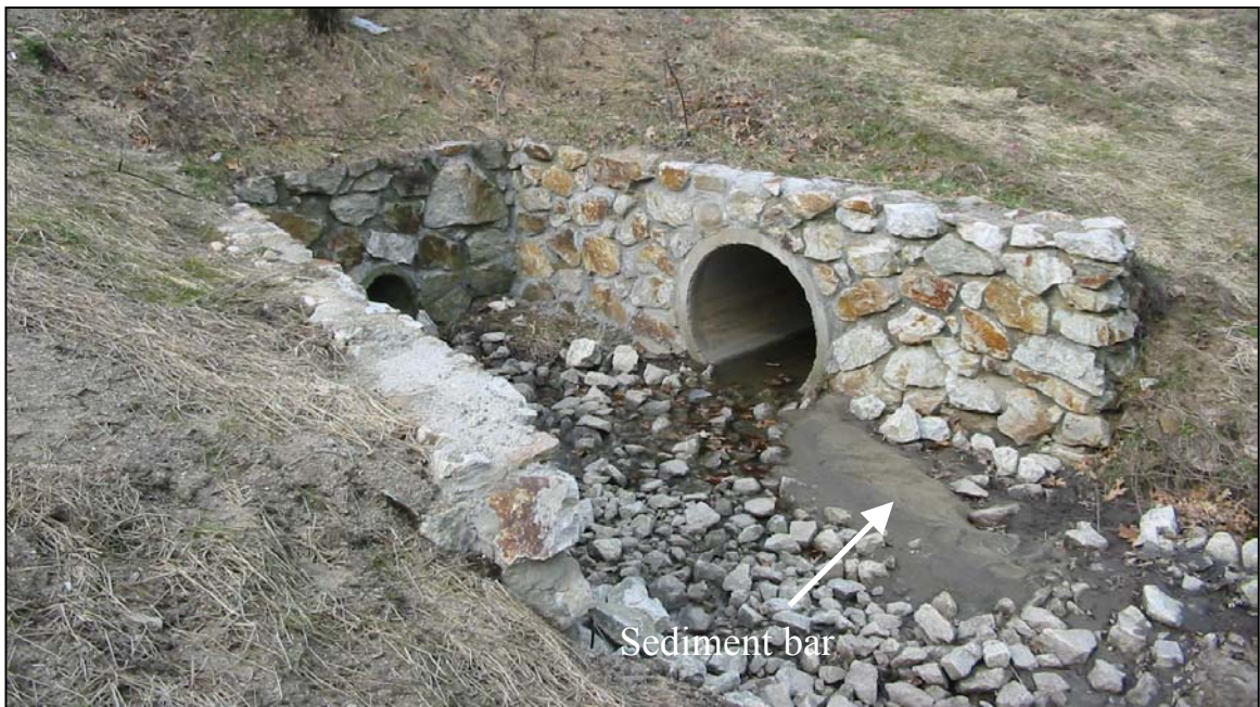
Figure 3-8. Route 101A 24" Discharge Pipe
