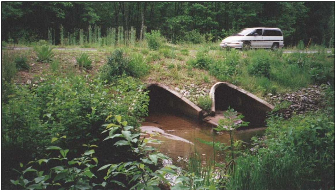
Figure 2-6. Stump Pond Brook Crossing under Seaverns Bridge Road
