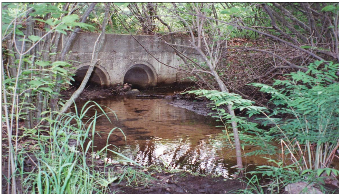
Figure 2-4. Bates Road Tributary Passing under Hansom Drive
