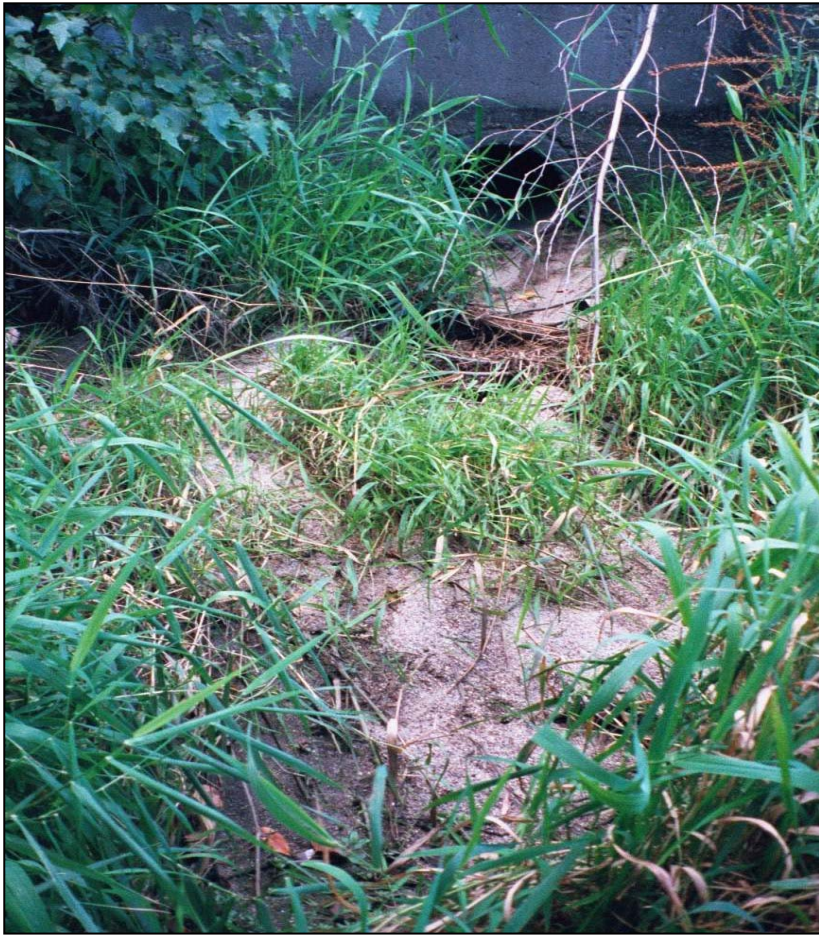
Figure 2-30. The outlet discharges into the wetland area.
