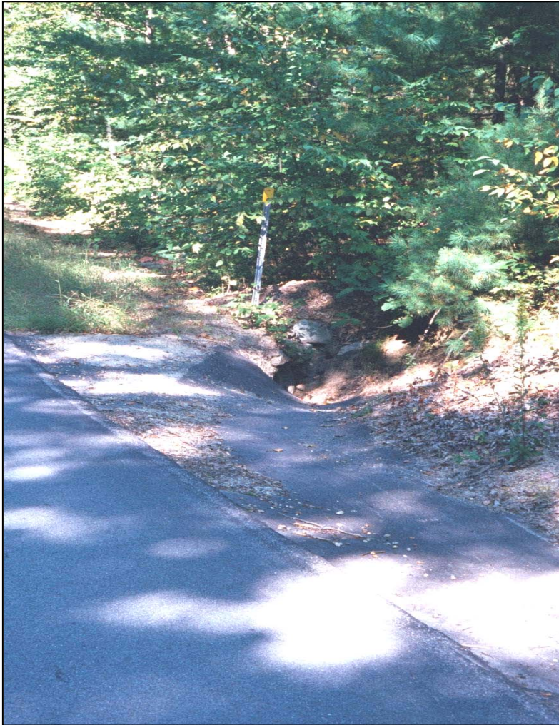
Figure 2-15. A paved swale along the eastern side of Rocky Hill Road.
