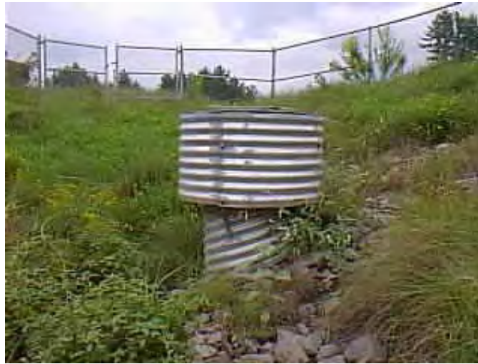
Figure 4. DOT Retention Basin Outlet (overflow)
