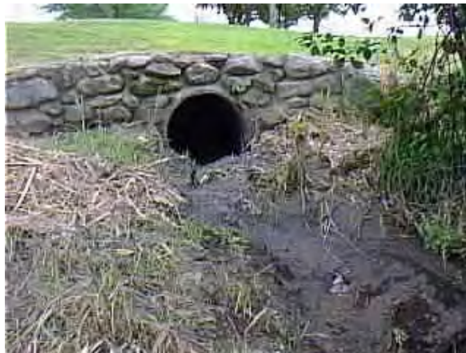
Figure 5. Somerset Plaza Swale Inlet
