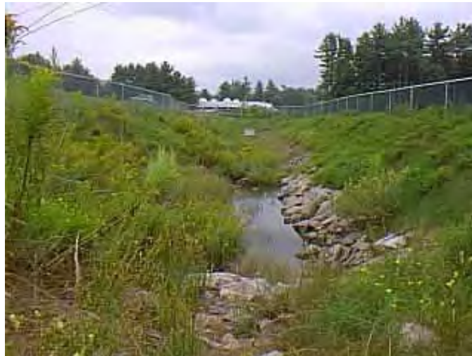
Figure 3. DOT Retention Basin Inlet
