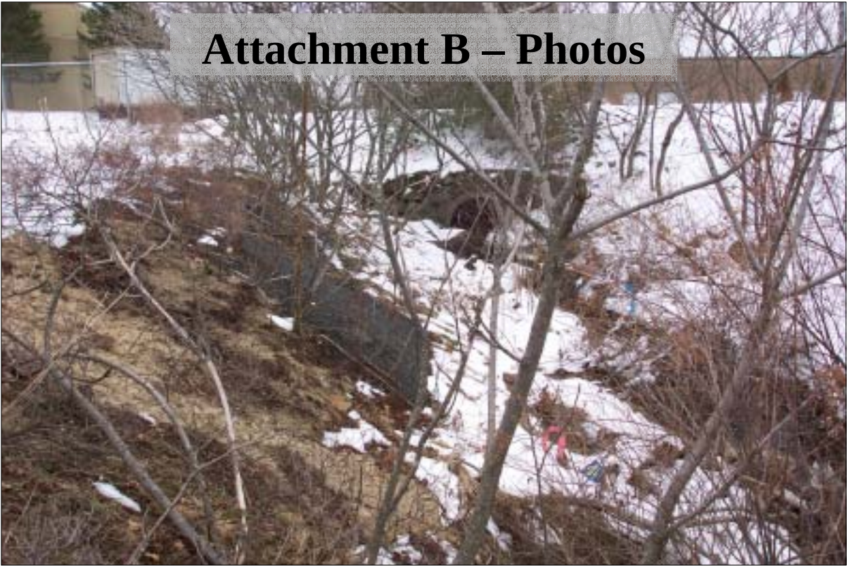
View of Discharge Outlet into Ditch from Celina Avenue
