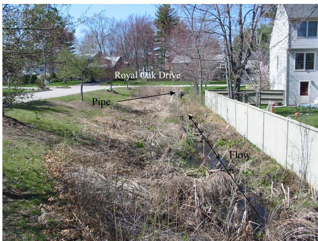
Figure 2-11 Unnamed Tributary before Being Channeled Underground for \frac{1}{3} Mile PBS, PBH, PBP, WBS, and MB Subwatershed Study Pennichuck Water Works
