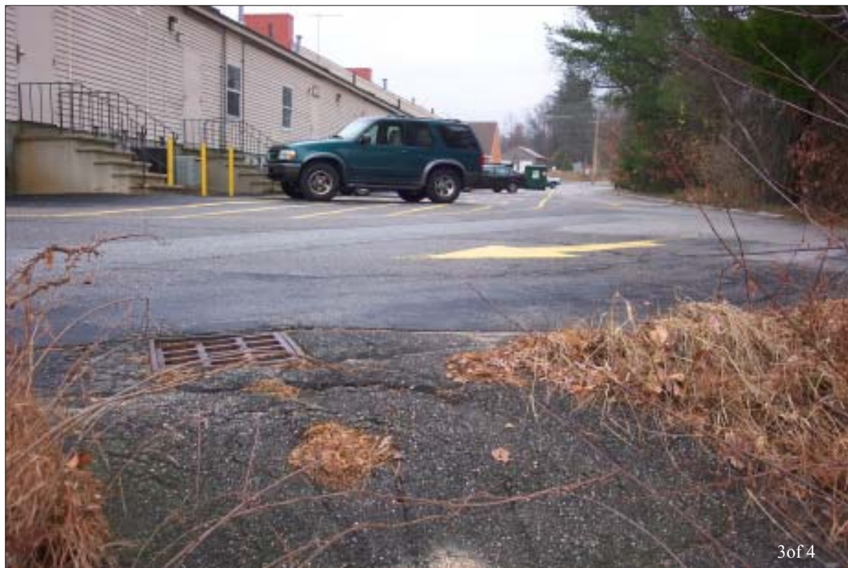
View of Access Road Behind Plaza – Catch Basin in Foreground
