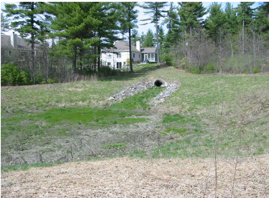
Figure 2-2 Functional Detention Basin for Heron Cove Housing Development
