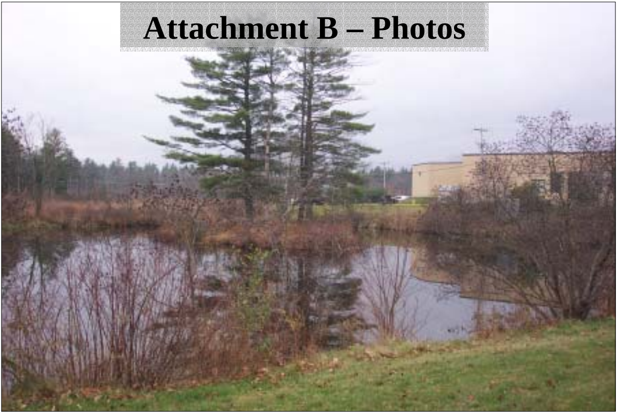
View of Detention Pond with the PC Connection Building in Background
