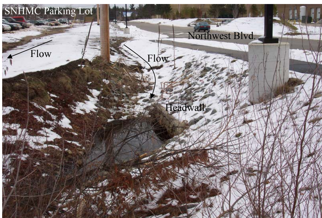
Figure 3-18 Aboveground Drainage Channels in Place of Catch Basins Provide Pretreatment for a Portion of Northwest Boulevard Runoff
