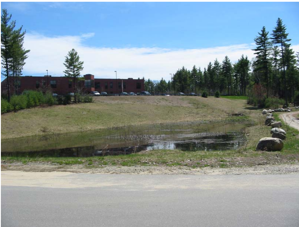
Figure 2-3 Functional Detention Pond at Heron Cove Office Park
