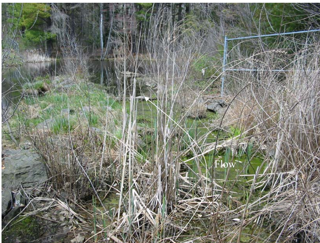
Figure 2-18 Weed Infested Channel at Harris Pond's Edge from Turnpike Discharge
