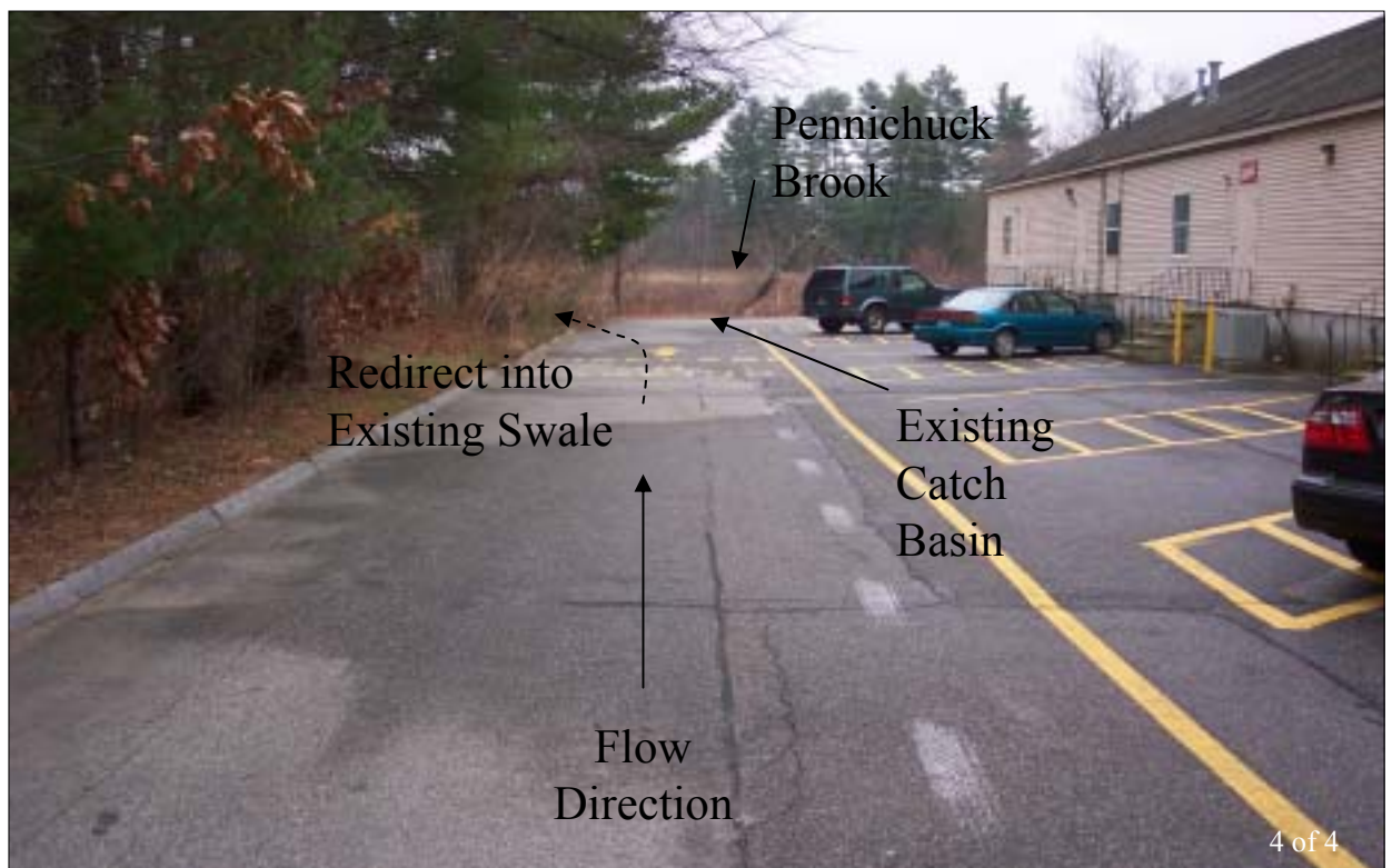
View of Access Road Behind Plaza
