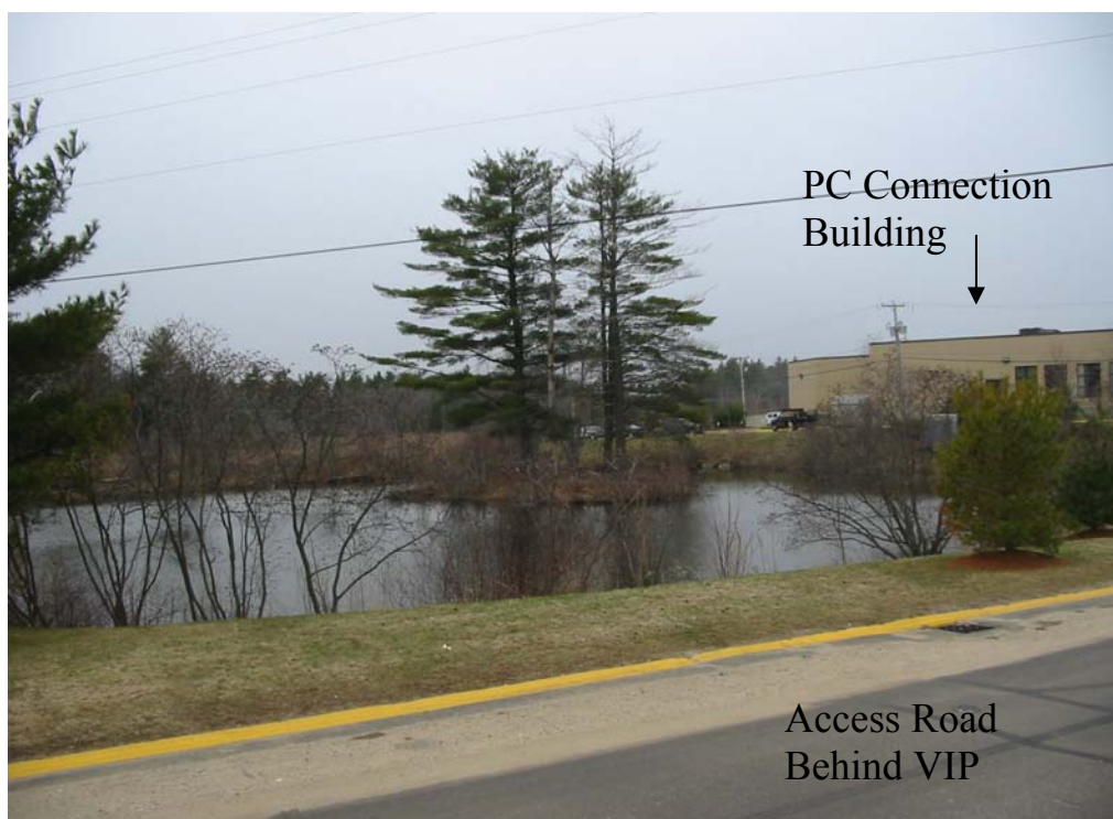
Figure 3-5 PC Connection Detention Pond Collects Runoff from Nearby Sites
