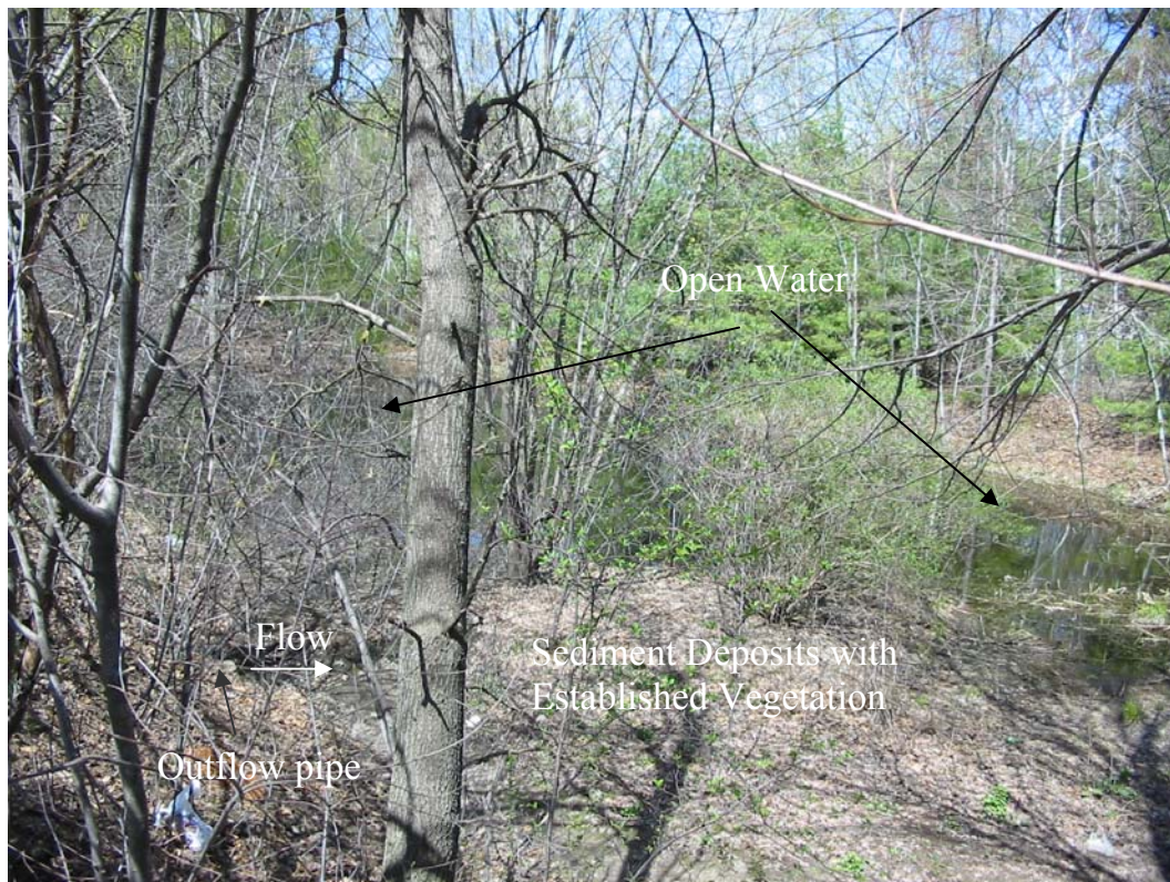
Figure 2-6 Sediment Filled Vespa Lane Detention Pond
