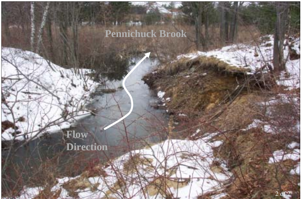
View of the End of the Drainage Ditch– Note major bank erosion on right
