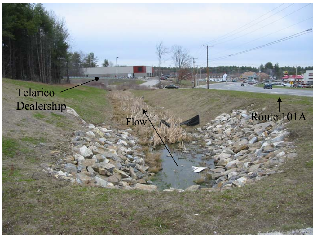
Figure 3-6 Vegetated Swale Near Home Depot Entrance Treats Site Runoff
