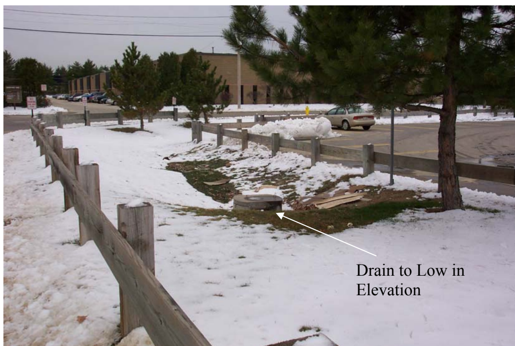
Figure 3-14 Marginally Effective Infiltration Swale behind The Mill Store
