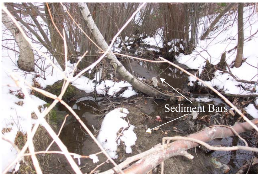
Figure 3-28 Accumulated Sediment in Channel from Westside Plaza Parking Area
