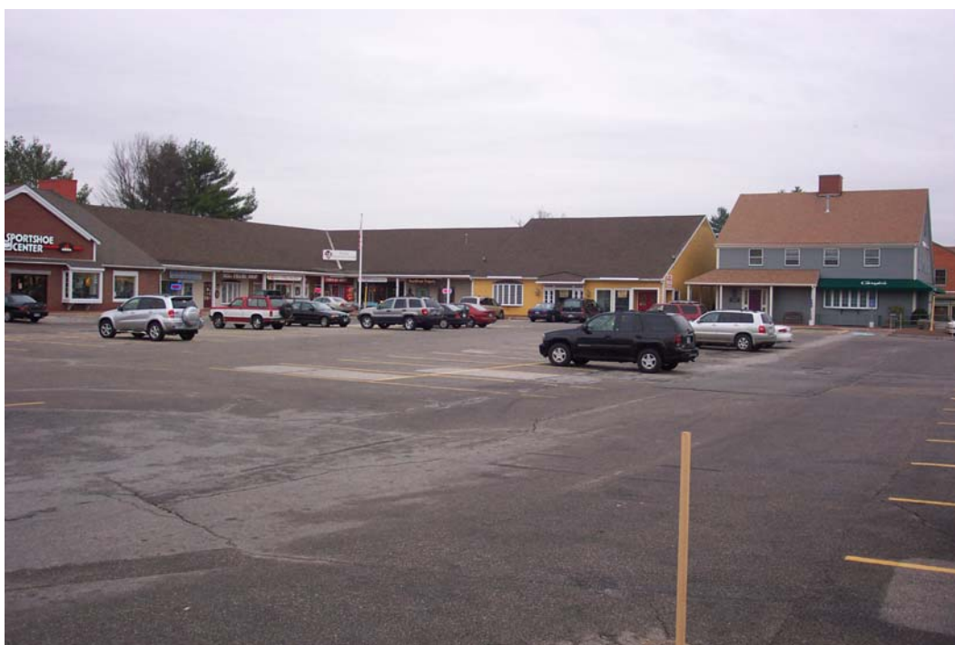
Figure 3-8 No On-Site Stormwater Treatment at Pennichuck Square Plaza
