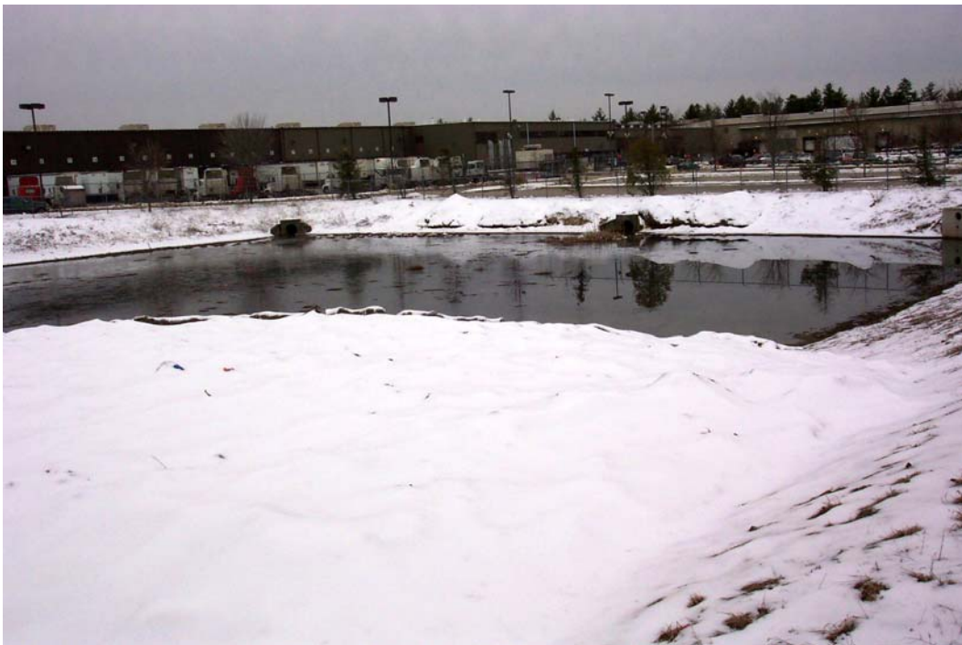
Figure 3-15 U.S. Postal Facility's Detention Pond Capturing Runoff from Site
