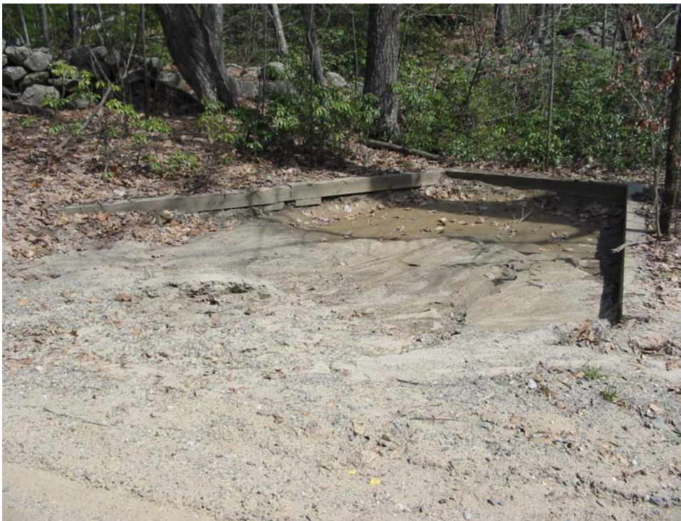
Figure 4-3 Working Sediment Trap on Federal Hill Road
