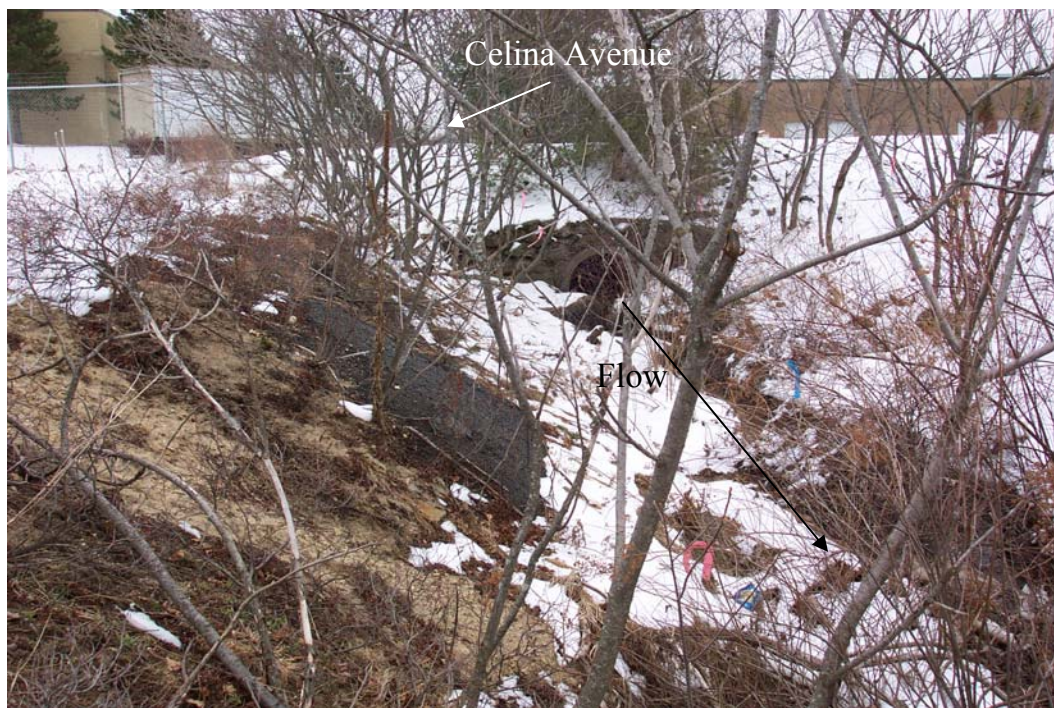
Figure 3-13 High Velocity Discharge from Celina Avenue Causes Scouring and Downstream Sedimentation
