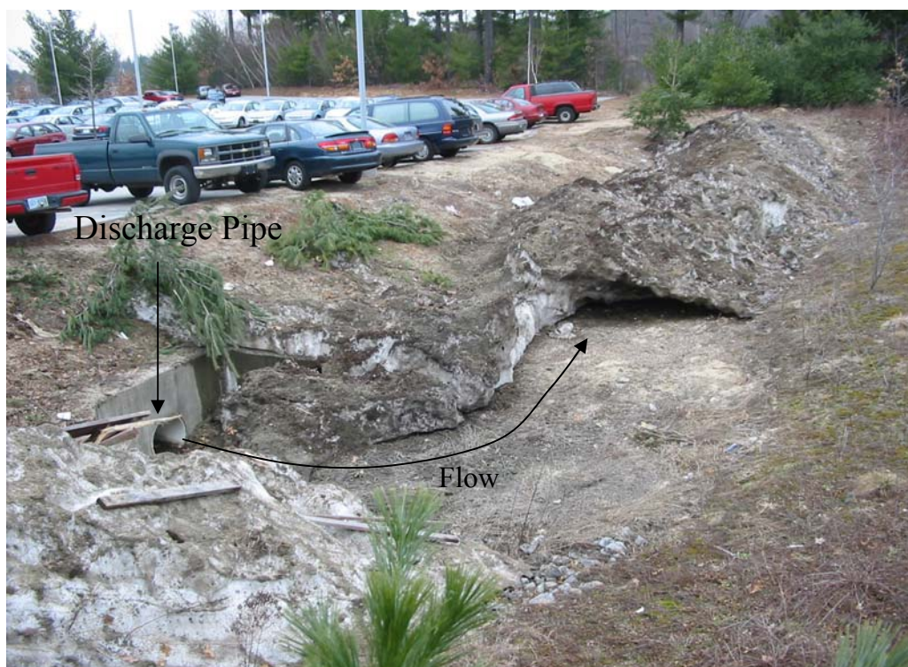
Figure 3-11 Functional Infiltration Basin Behind Saturn Dealership
