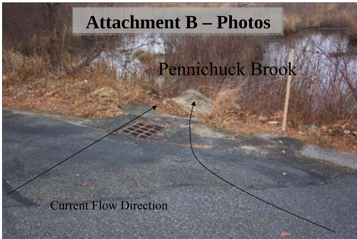
Close-up View of Paved Drainage Swale and Catch Basin Located Behind the Plaza
