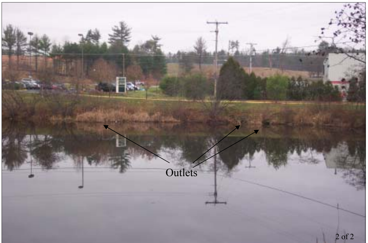
View of Three Partially Submerged Discharge Outlet Pipes ( Outlets hidden behind vegetation) Flowing into the Detention Pond
