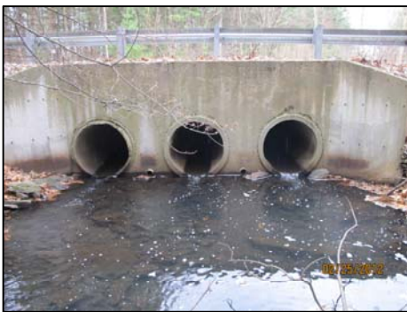
Culvert Crossing of Boire Field Brook at Tinker Road
