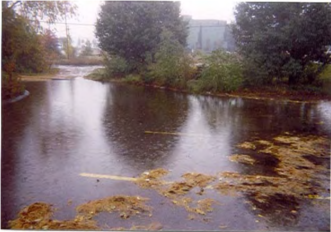
Figure 4-1. Ponding Problem at Sullivan Tire
