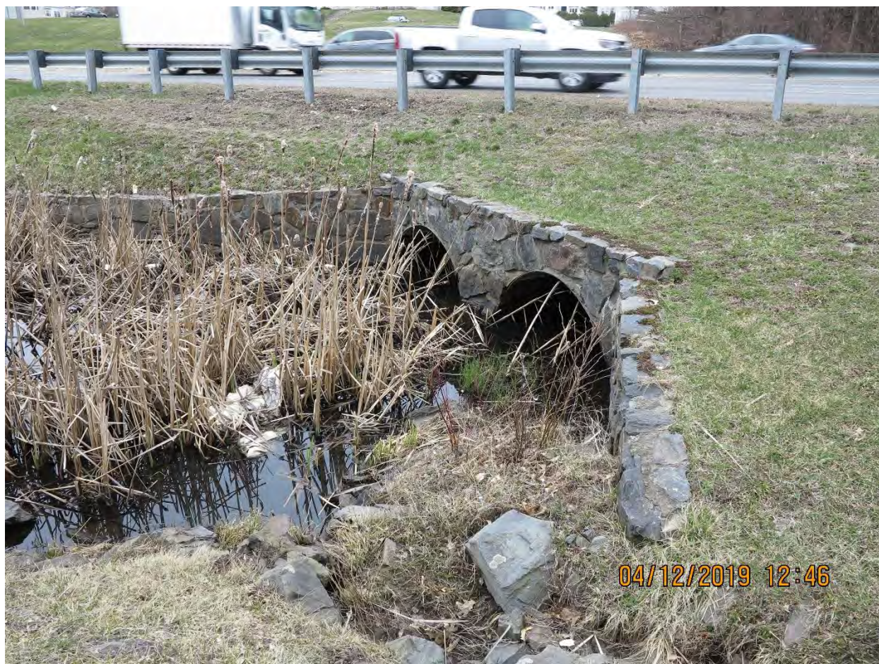
Corridor Site 1: Somerset Parkway culvert inlet from Somerset Parkway Swales (south side of crossing)
