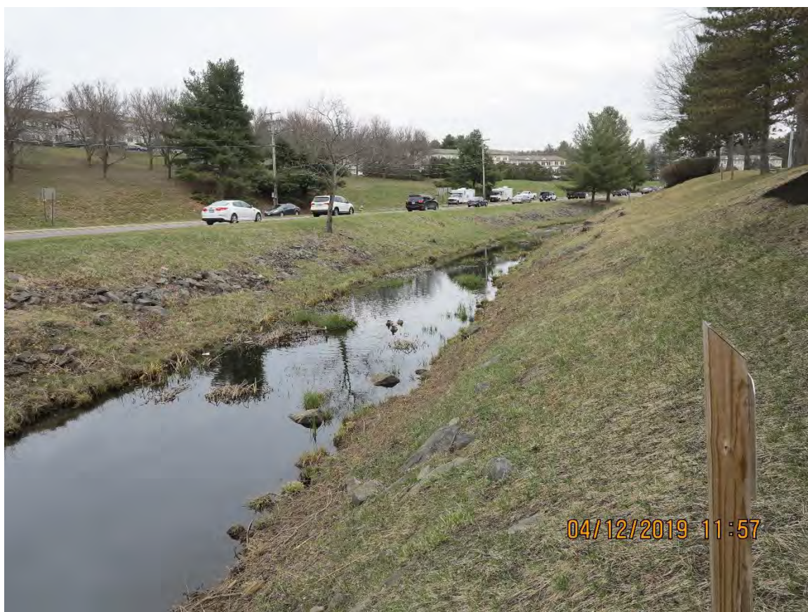
BMP SITE 4: Somerset Parkway Swales
