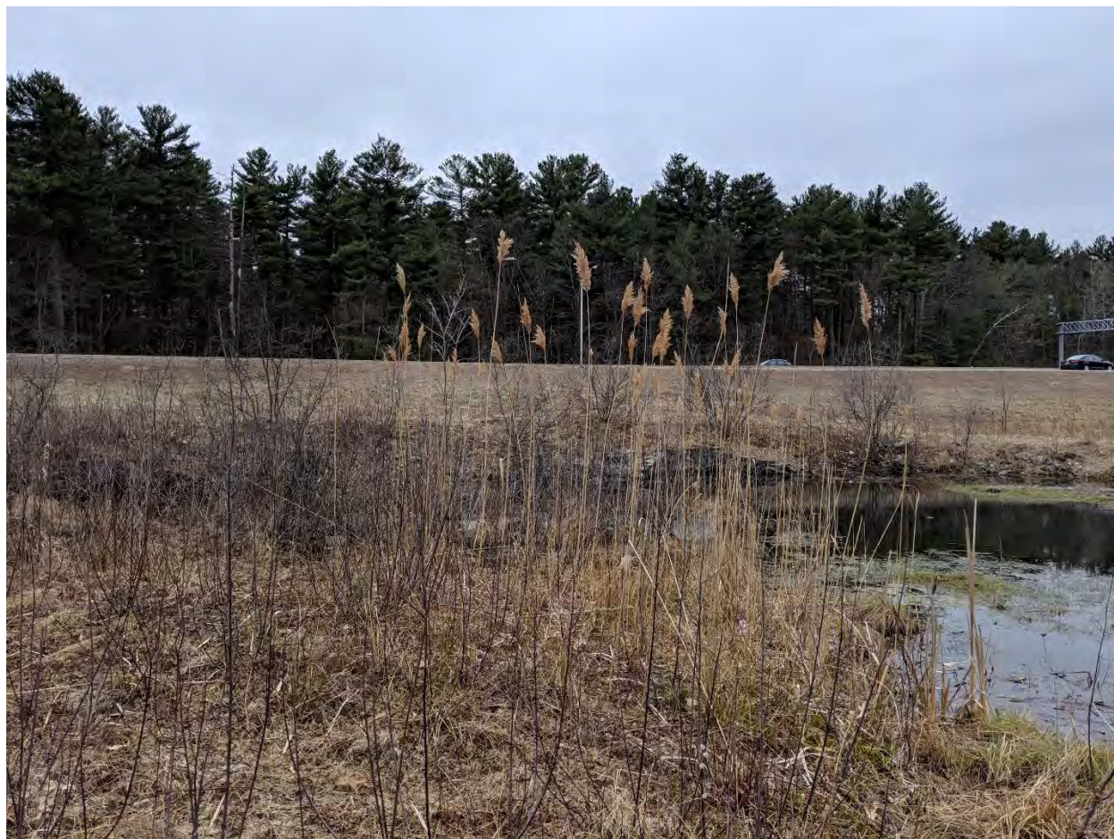
Corridor Site 16: Everett Turnpike culvert outlet (east side of crossing)
