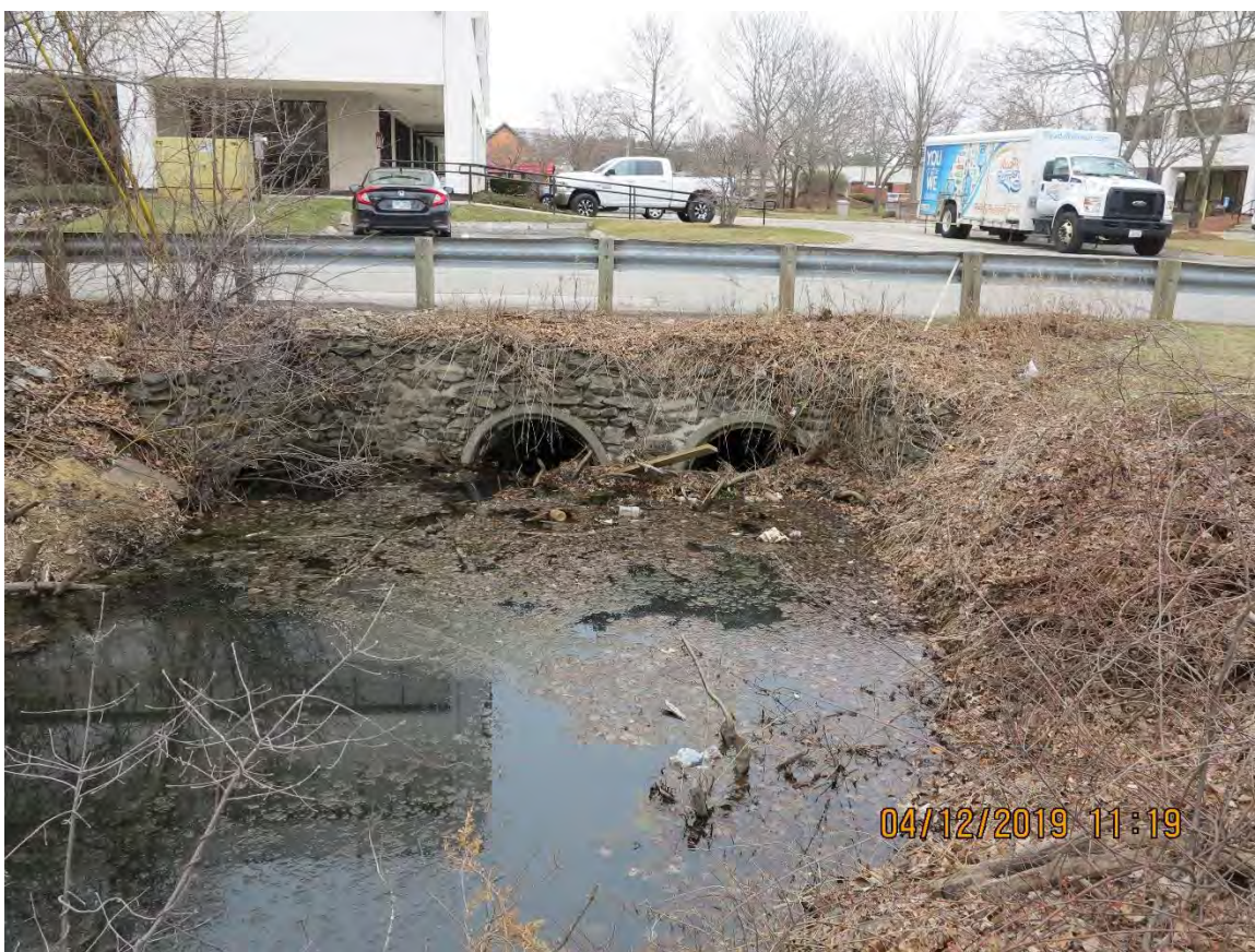
BMP SITE 2: Birch Pond Discharge Channel
