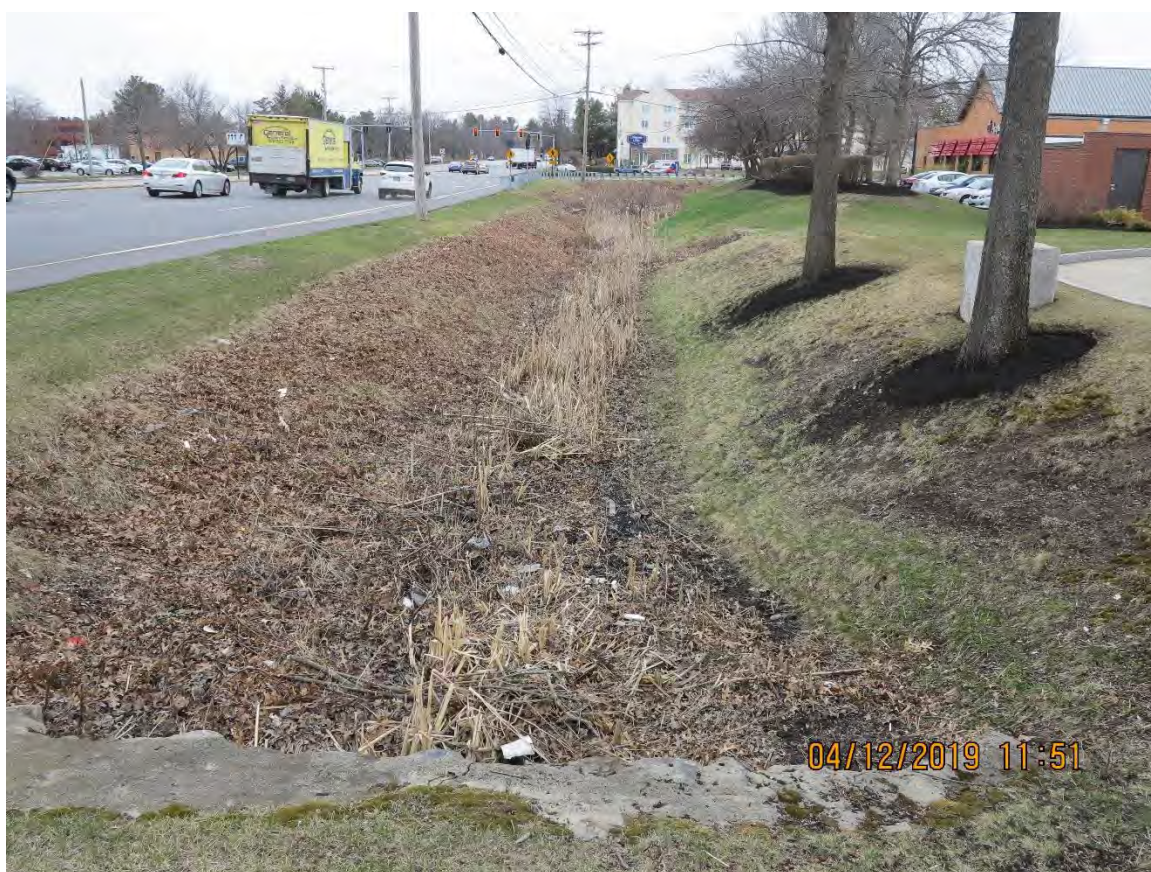
BMP SITE 4: Somerset Parkway Swales
