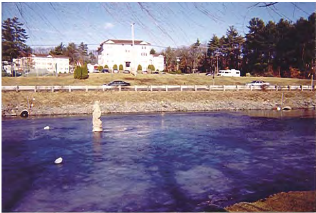
Figure 2-5. Stormwater Discharges to Crowne Plaza Detention Pond
