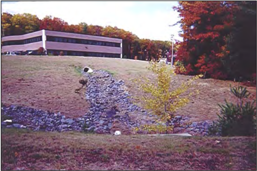
Figure 2-18. Stormwater Collection Junction for the Cornerstone Site
