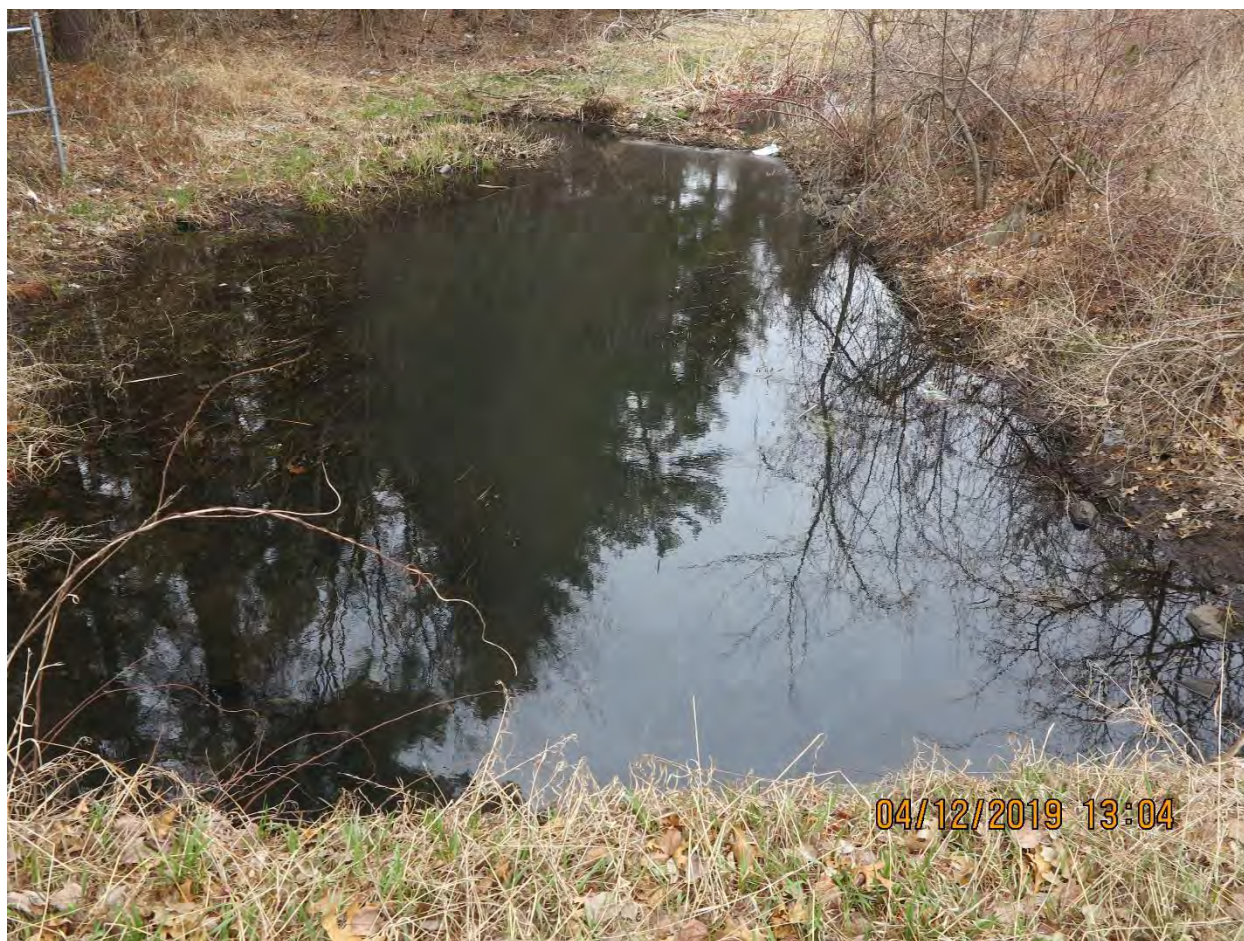
Corridor Site 2: Somerset Parkway culvert outlet (north side of crossing)
