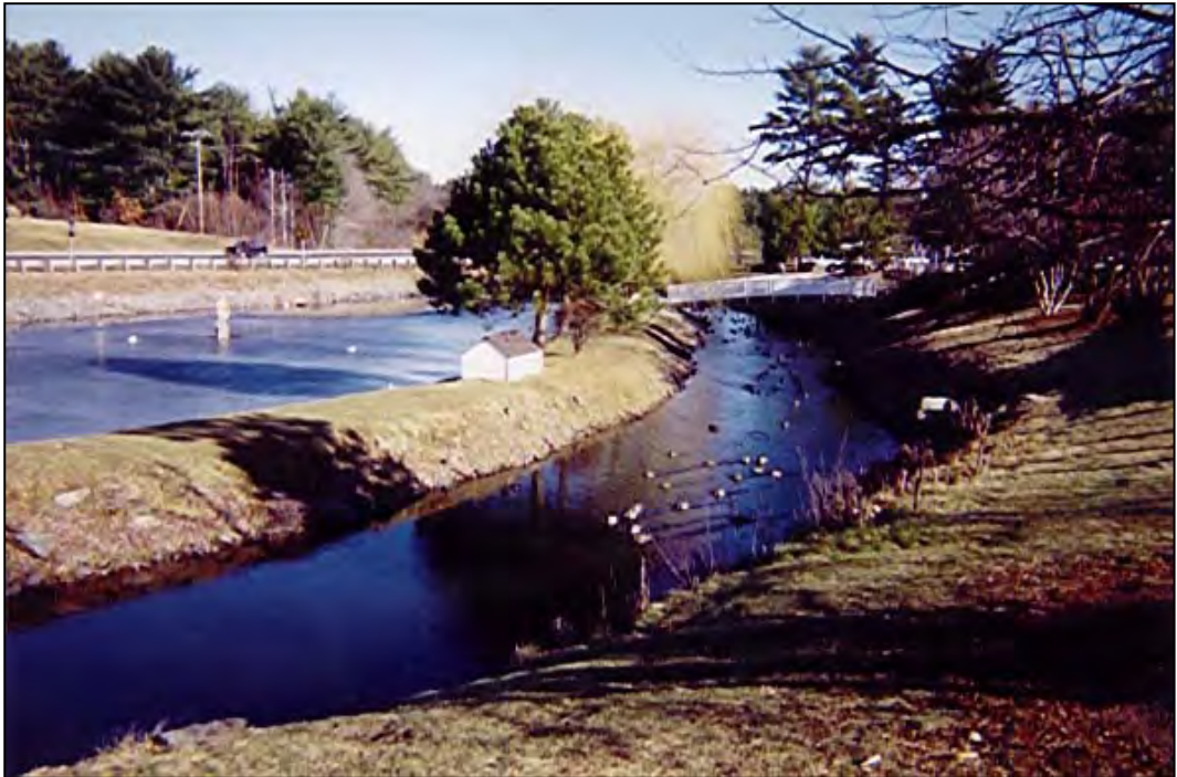
Figure 2-10. Crowne Plaza Detention Ponds
