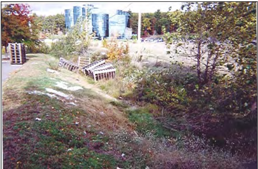
Figure 2-9. Northern Perimeter Swale
