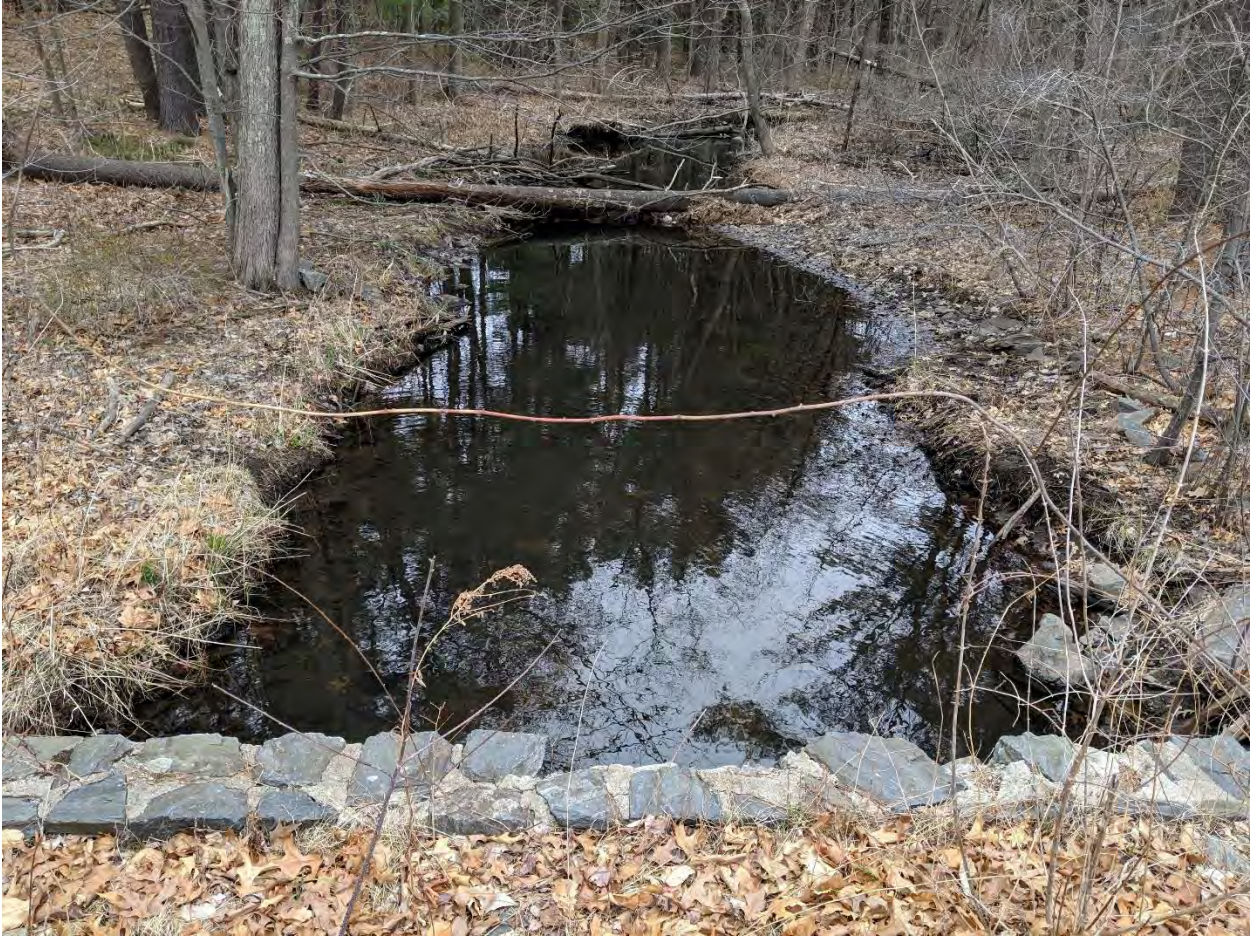
Corridor Site 4: North Southwood Drive culvert outlet (east side of crossing)
