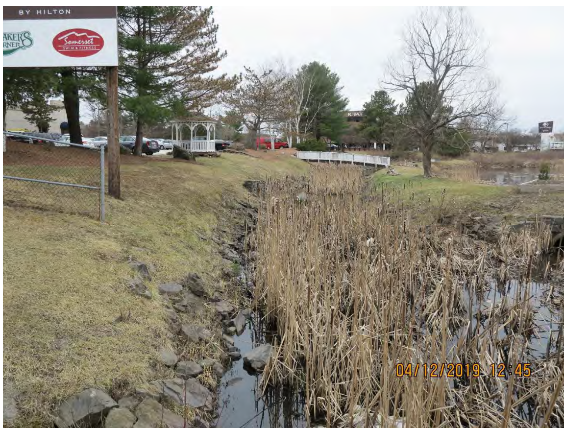
BMP SITE 4: Somerset Parkway Swales
