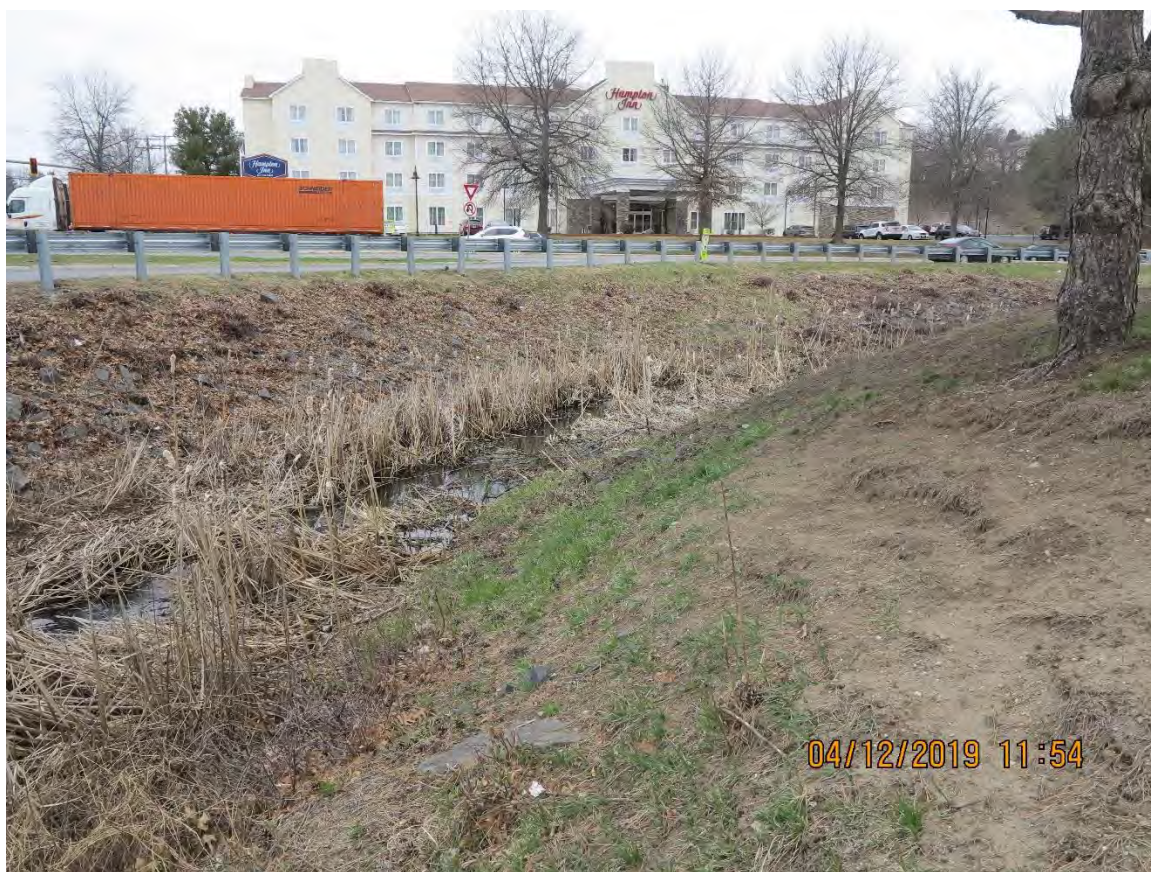
BMP SITE 4: Somerset Parkway Swales
