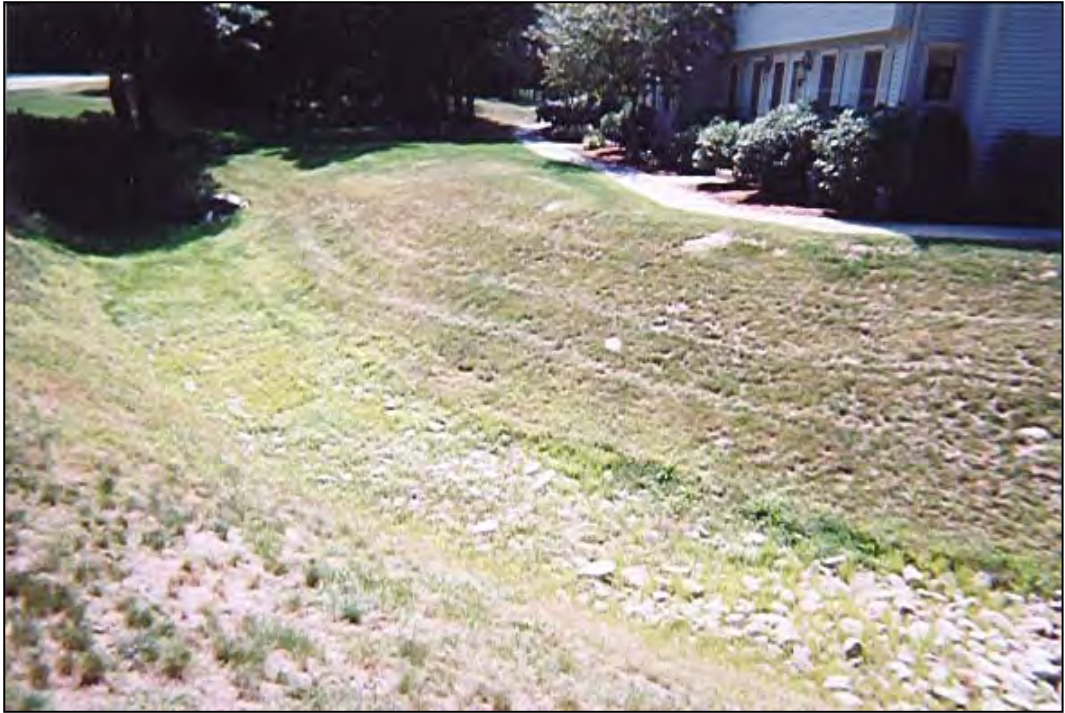
Figure 2-2. Kessler Farm Swale
