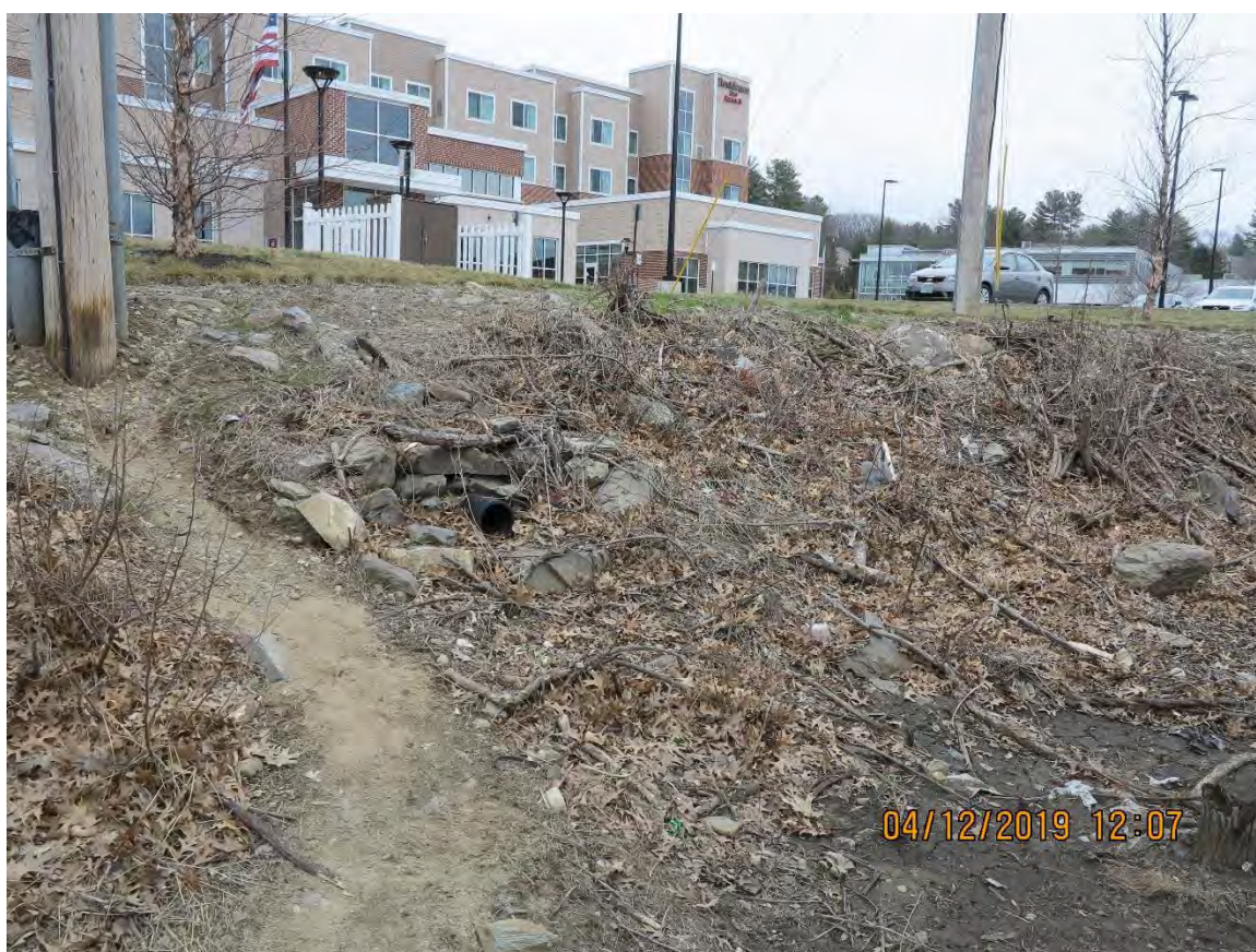
BMP SITE 6: Somerset Plaza Perimeter Swale
