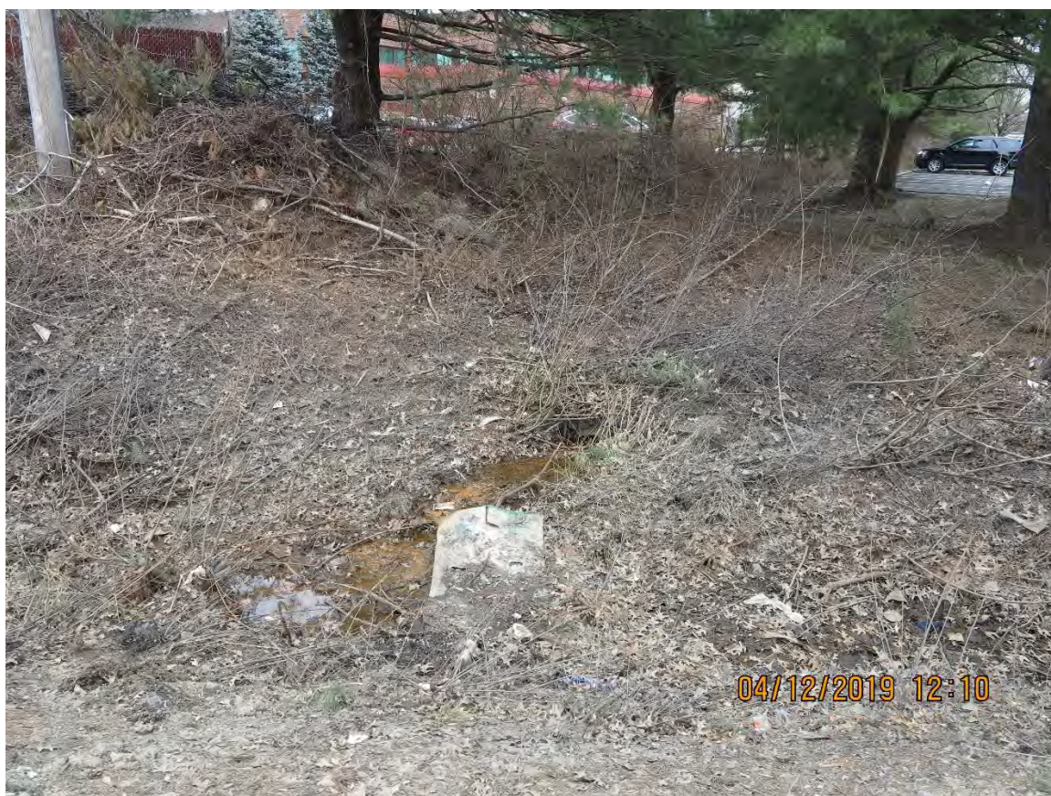
BMP SITE 6: Somerset Plaza Perimeter Swale
