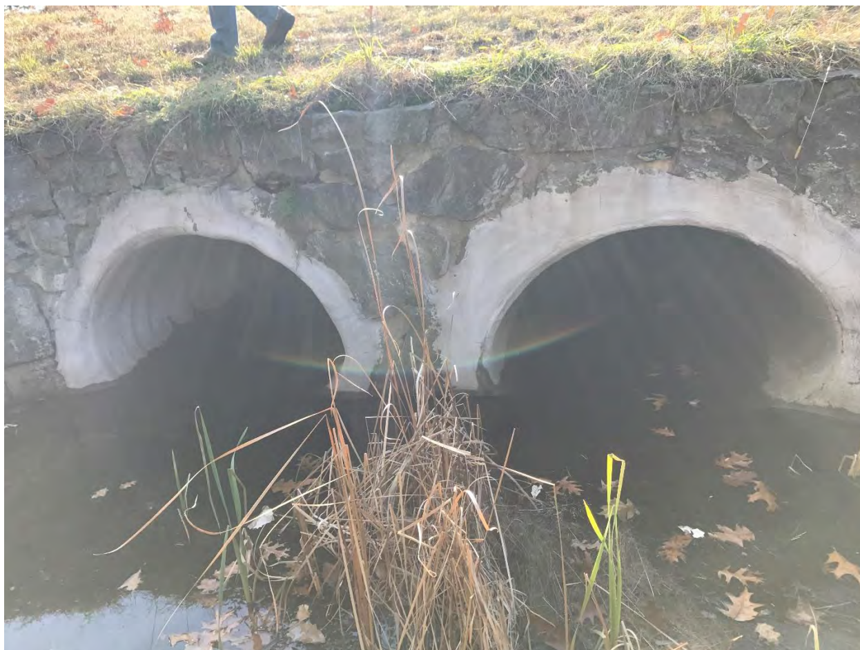
Corridor Site 5: North Southwood Drive On-Ramp culvert outlet from Somerset Parkway Detention Basin (north side of crossing)
