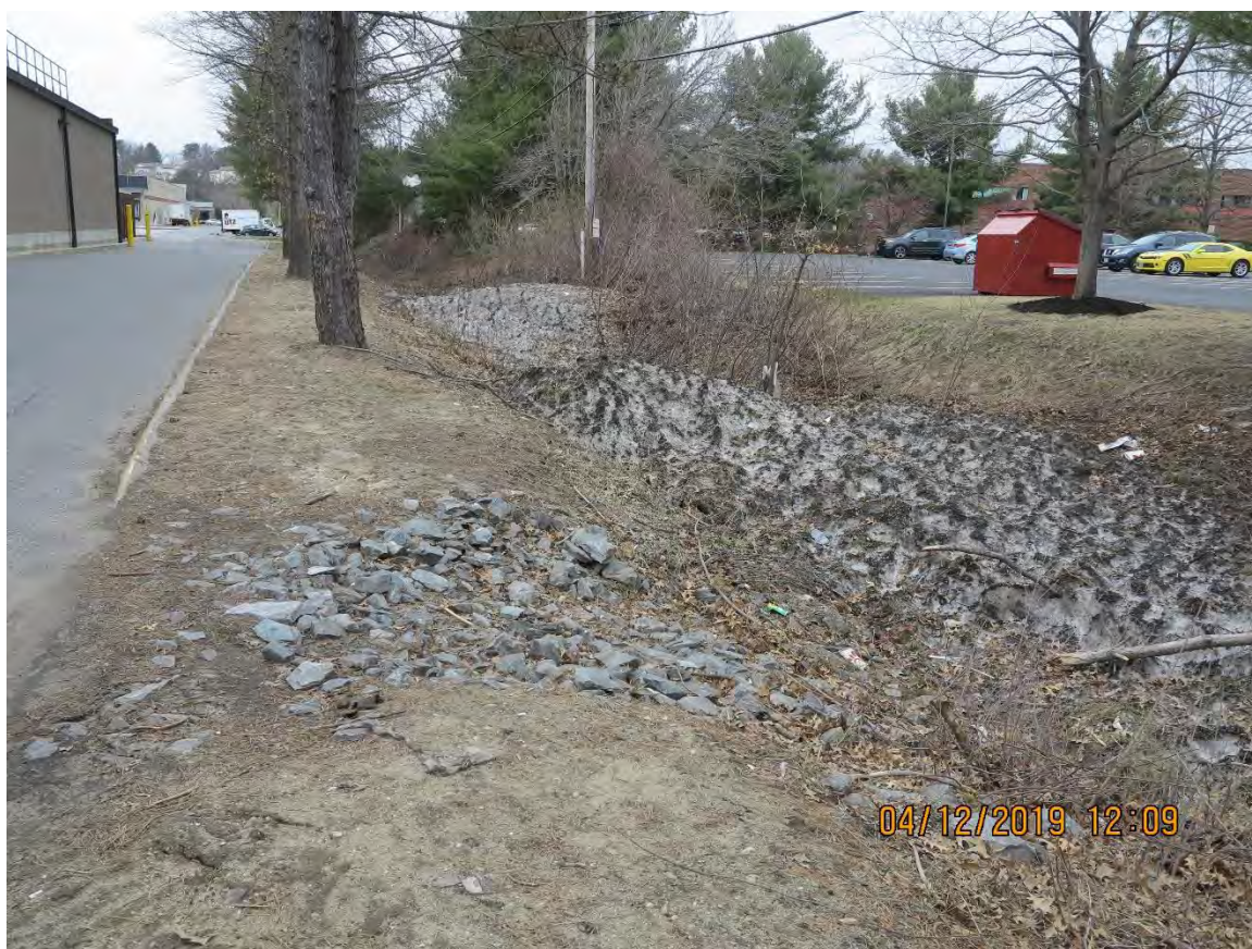
BMP SITE 6: Somerset Plaza Perimeter Swale
