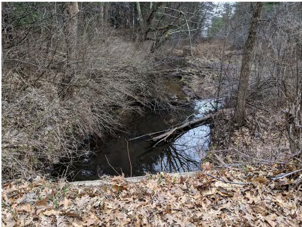
Corridor Site 8: Tinker Road culvert inlet (south side of crossing)
