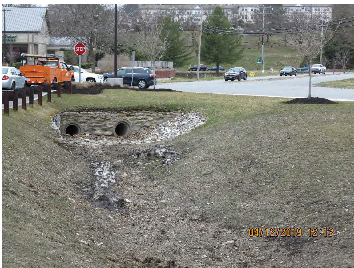
BMP SITE 6: Somerset Plaza Perimeter Swale
