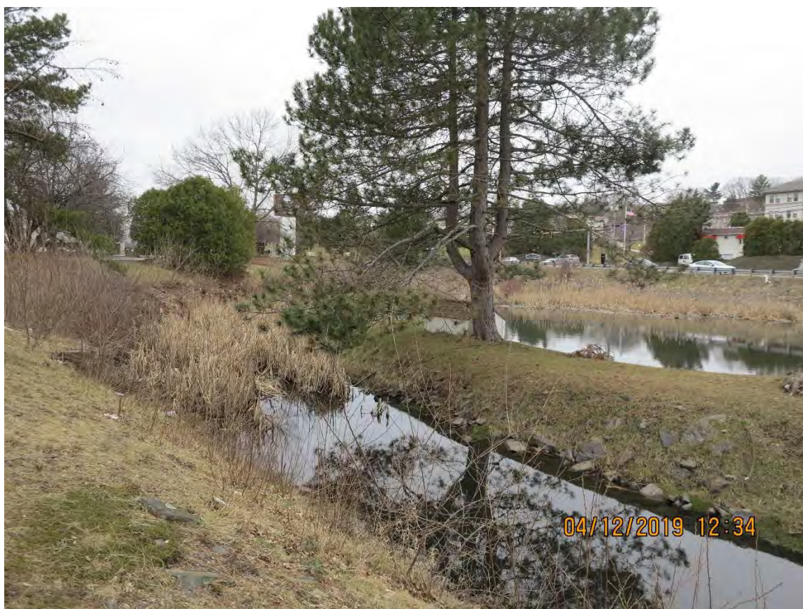
BMP SITE 4: Somerset Parkway Swales
