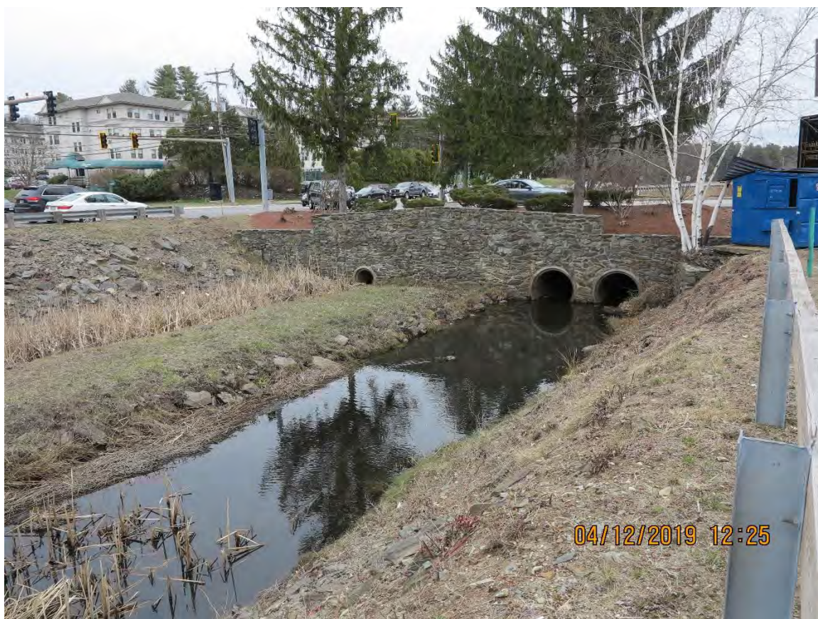
BMP SITE 4: Somerset Parkway Swales
