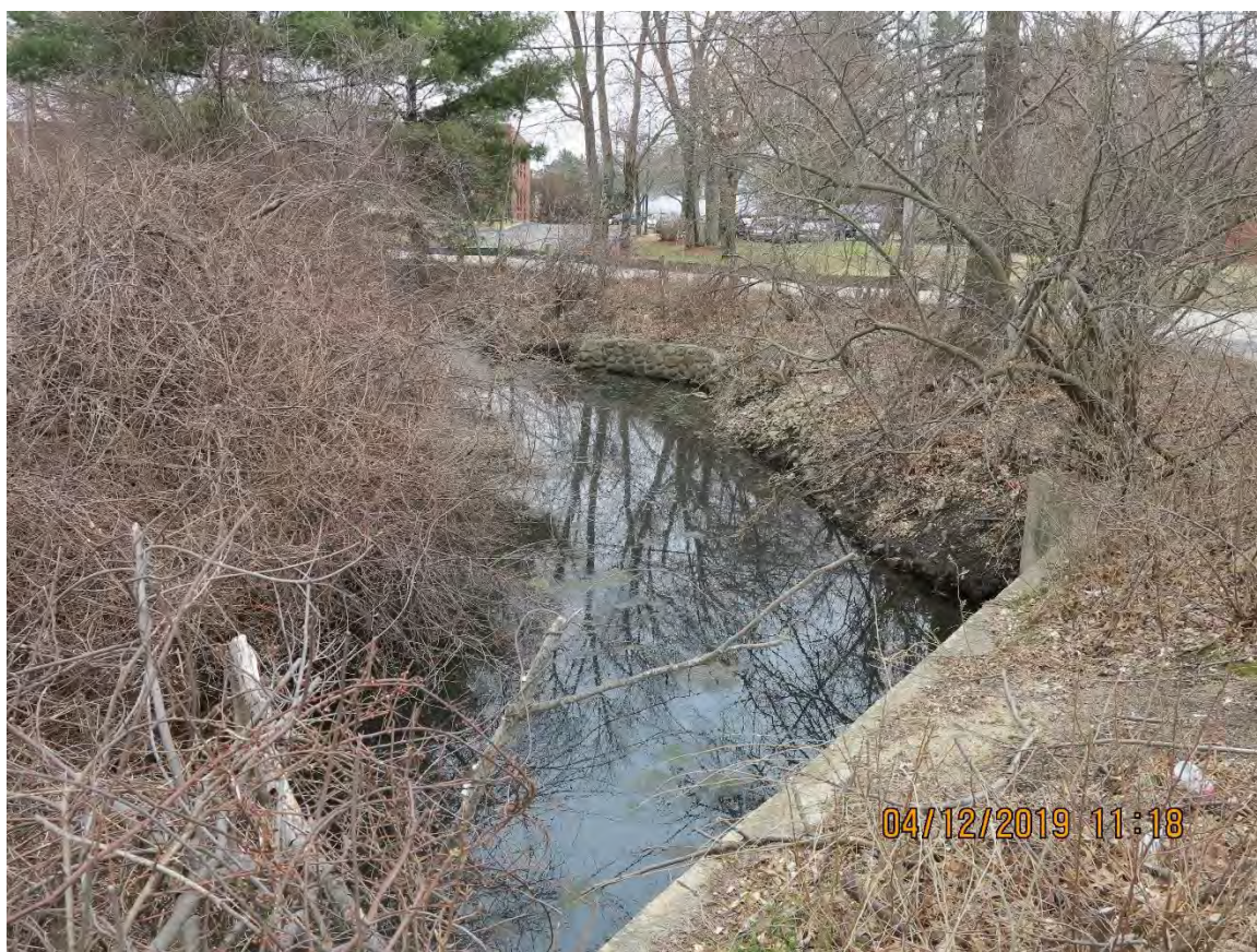
BMP SITE 2: Birch Pond/Birch Pond Discharge Channel
