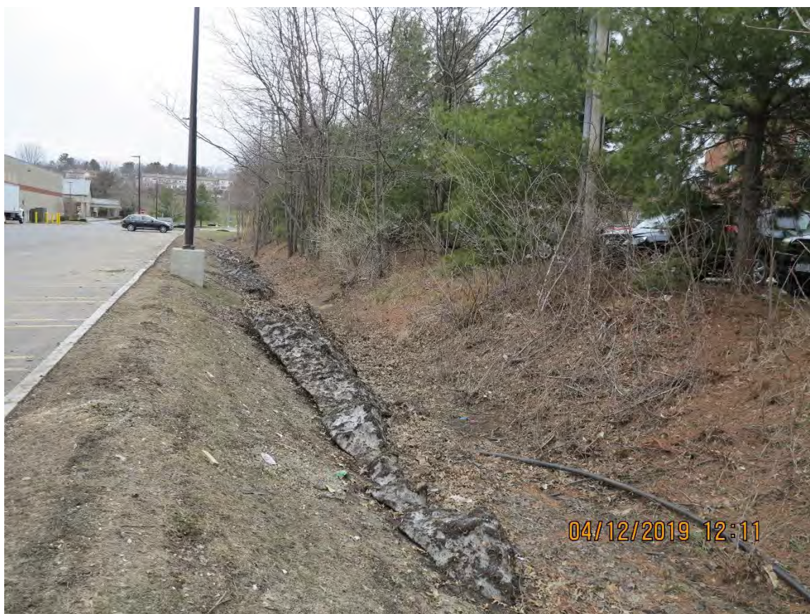
BMP SITE 6: Somerset Plaza Perimeter Swale
