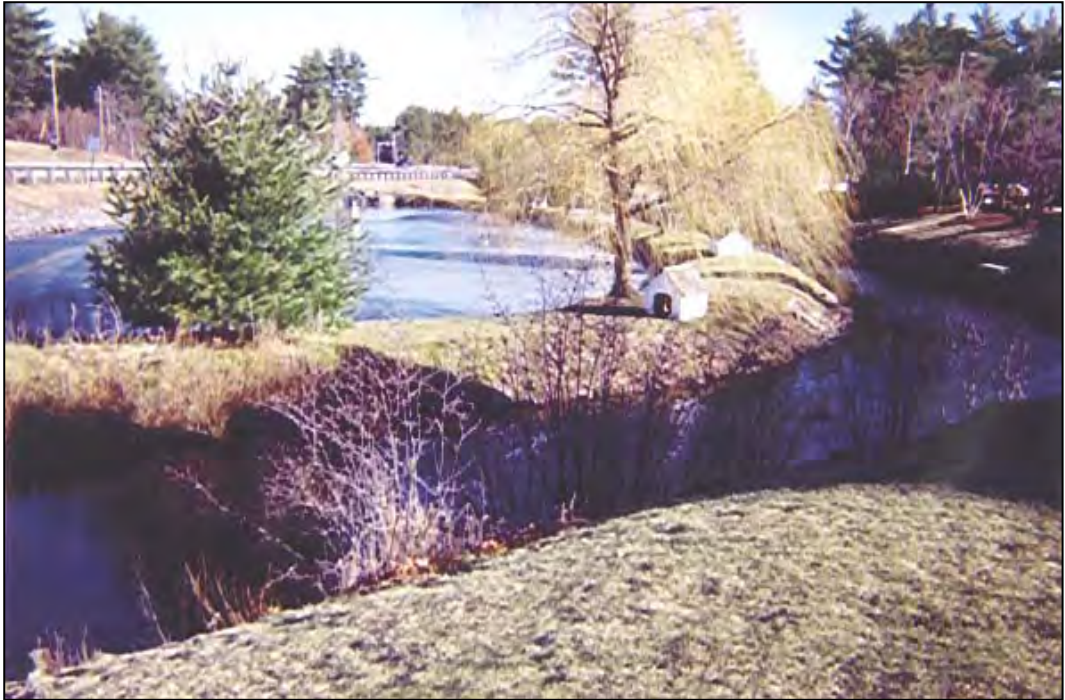
Figure 3-5. Crowne Plaza Detention Ponds
