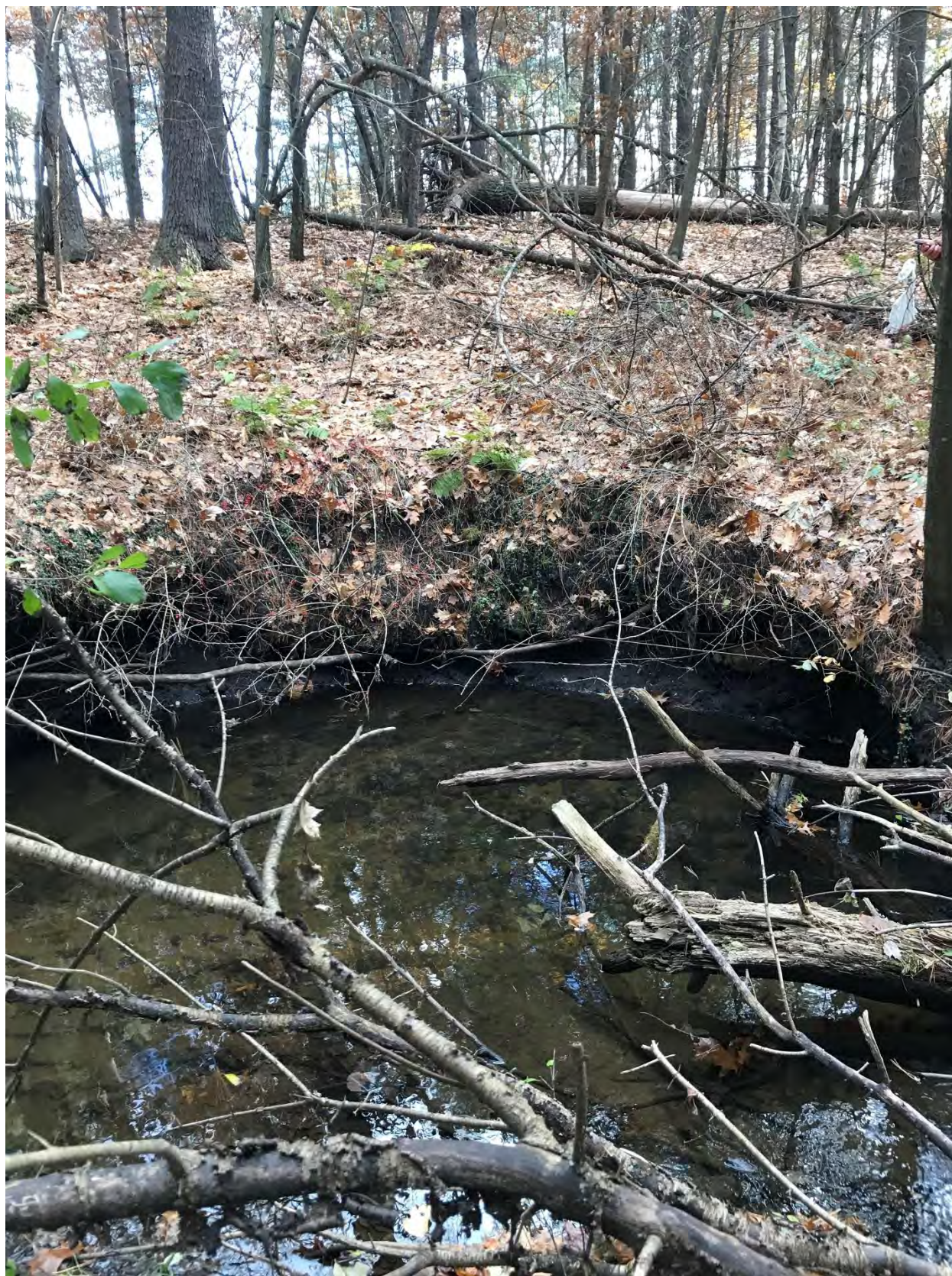
Corridor Site 12: Bank erosion and undercutting due to larger flows
