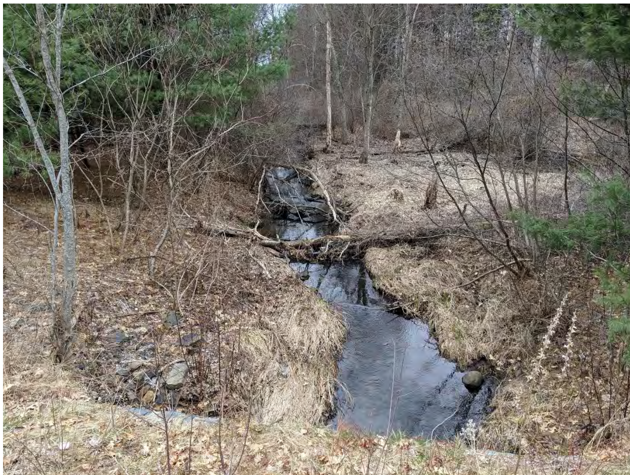
Corridor Site 3: North Southwood Drive culvert inlet (west side of crossing)
